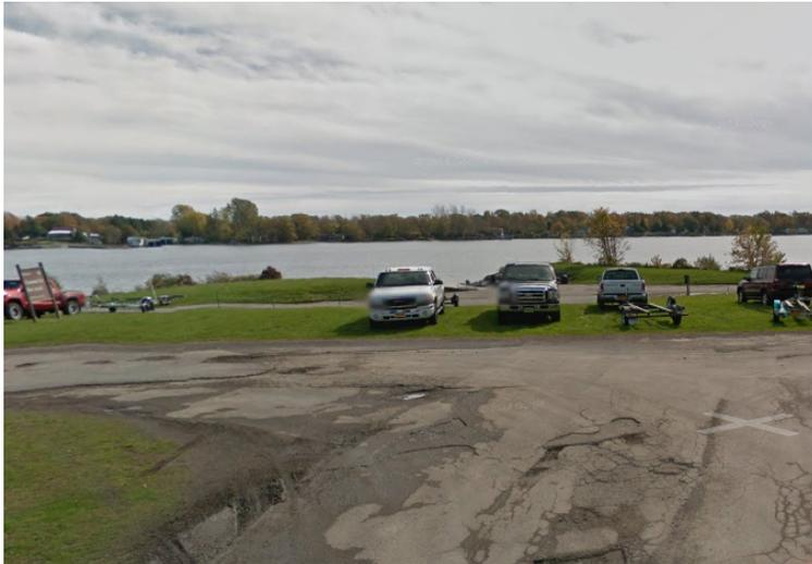
The drive isles and the parking area pavement at the boat launch is in poor condition and needs to be replaced.
